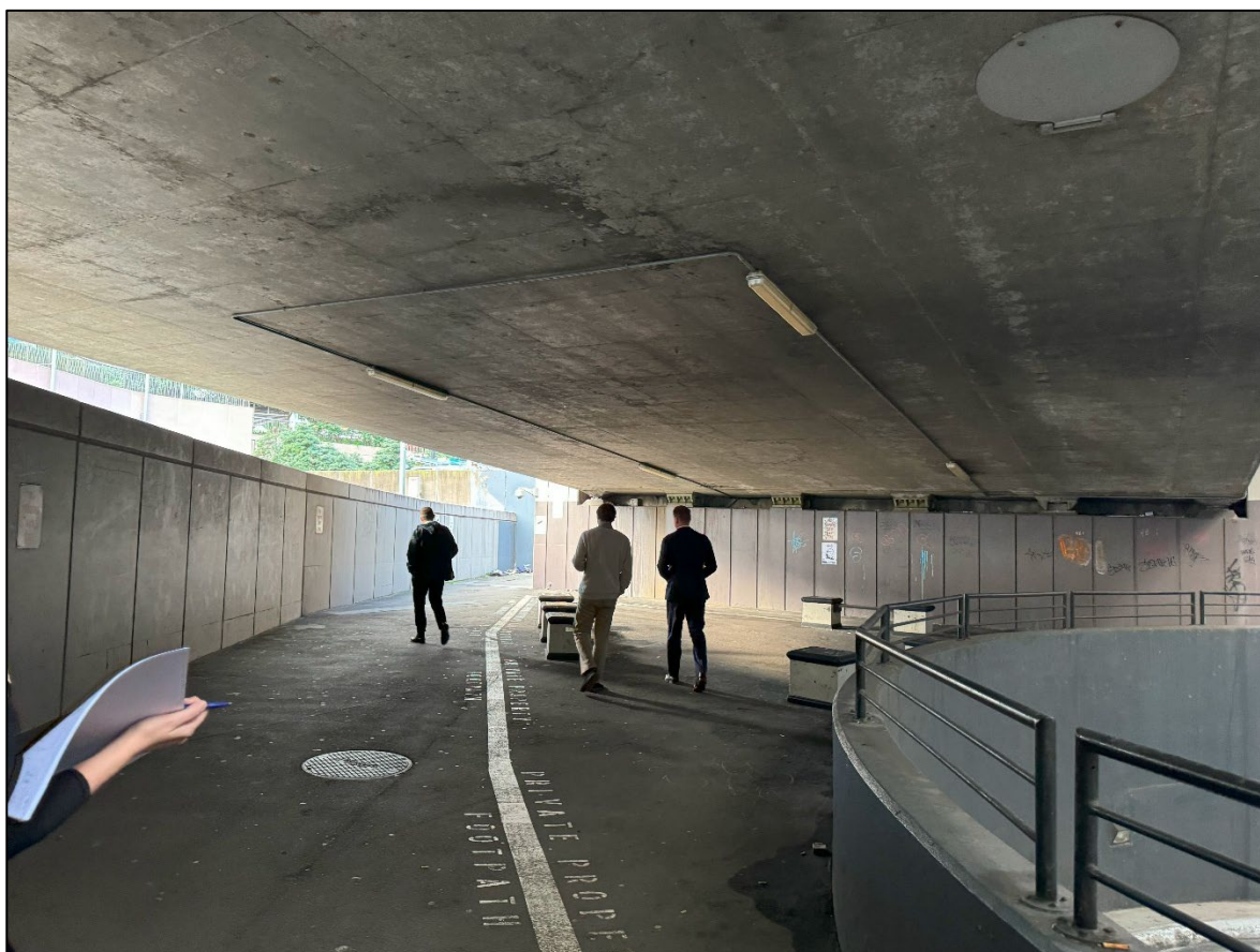
Figure 5 View north east of pedestrian link under Western Distributor Source: Hassell
